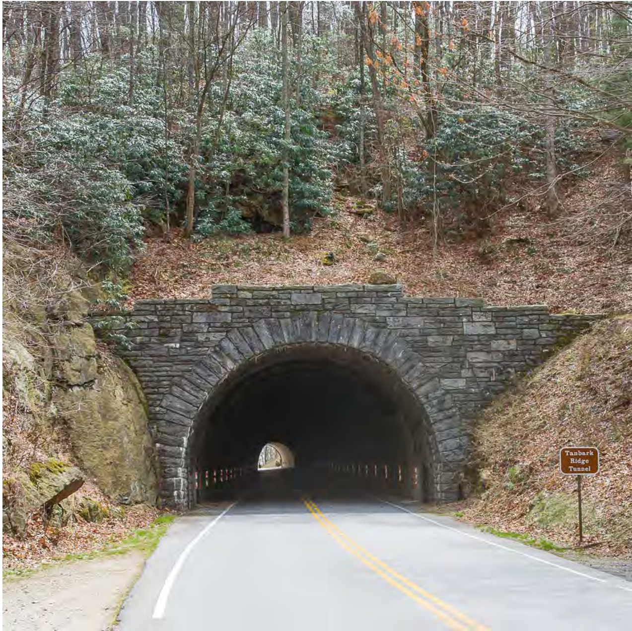
Blue Ridge tunnel - April 2007
