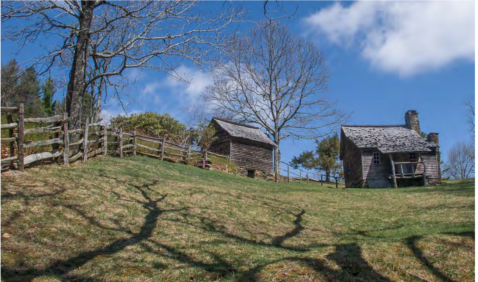
This cabin was lived in by the Brinegar family until 1935 when the parkway was built. - April 2007
