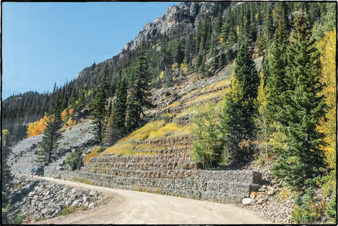
This hair-pin curve has been recently fortified so that the road doesn't wash out in heavy rain storms.
